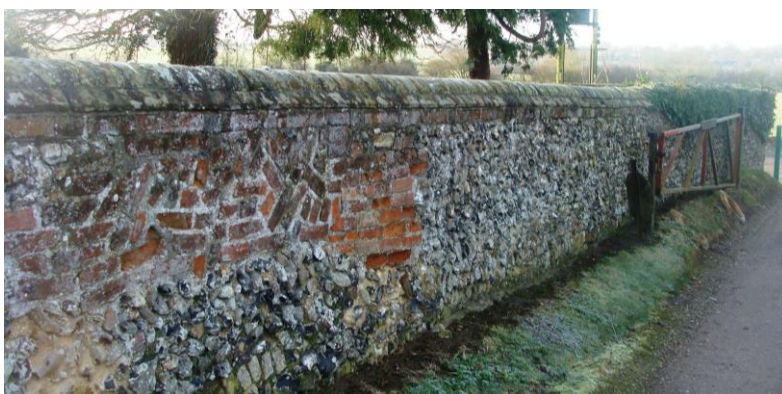
Picture 22. Good quality 19th century wall at High Hall Farm worthy of retention and protection.
